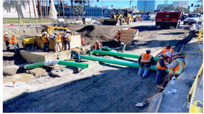
Street Restoration Work at Wilshire/Fairfax Station
