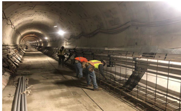
Reach 3 BL Tunnel Walkway Construction
