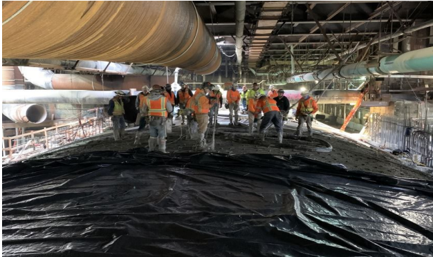
Last Roof Concrete Placement at Wilshire/La Brea Station
