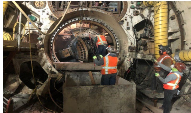
Reach 4 South Tunnel TBM Cutterhead Removal
