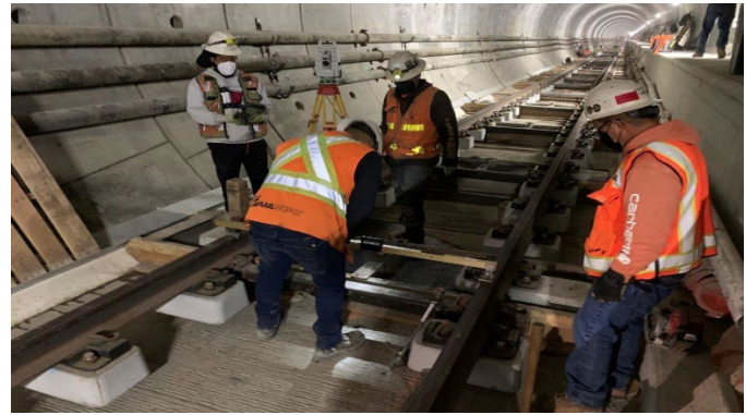
Reach 2 BR Tunnel Track Installation
