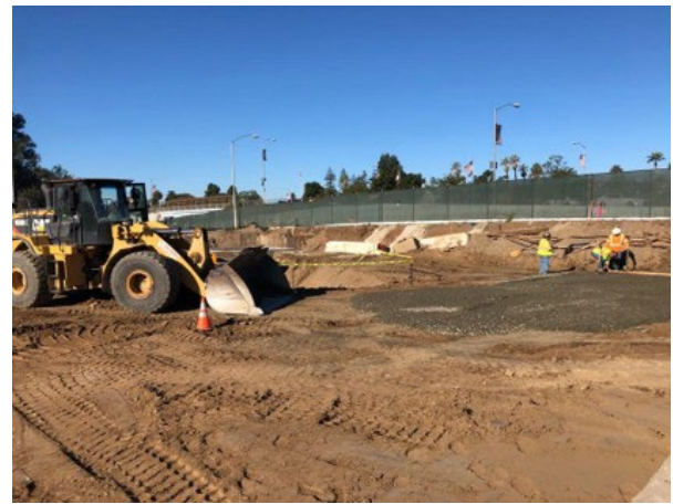
Backfilling of VA Steam Tunnel Redundant Line
