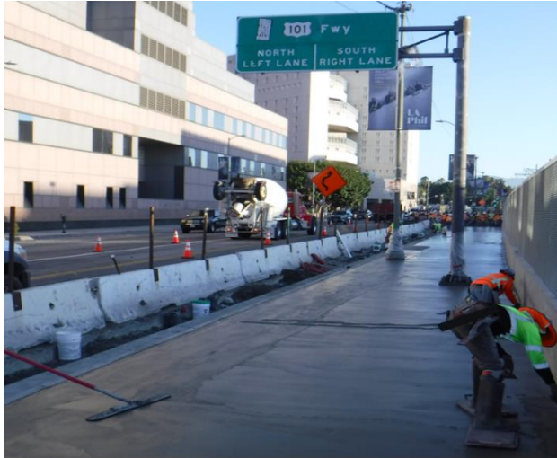
Concrete pour for Alameda sidewalk (between Temple and Commercial)
