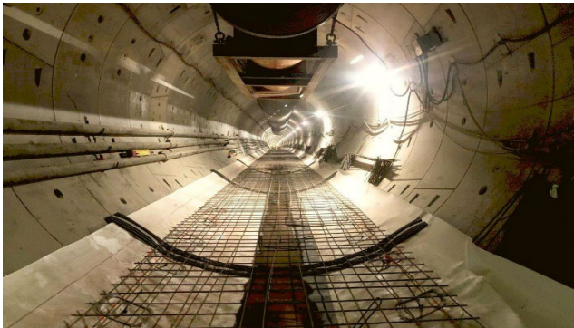
Reach 3 South Tunnel Invert Construction
