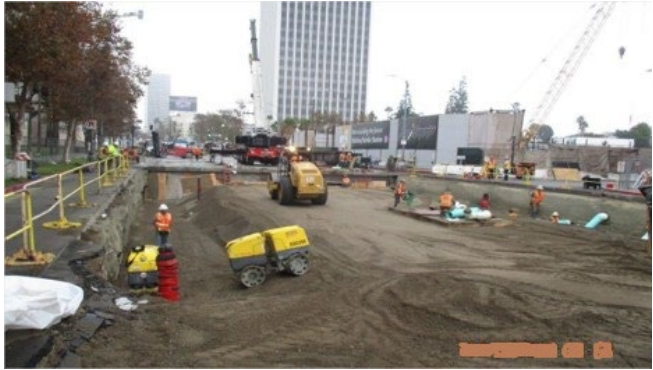
Street Restoration Work at Wilshire/Fairfax Station
