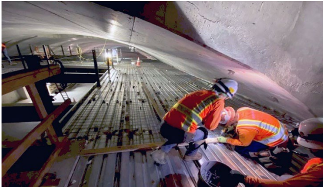
Plenum Construction at Wilshire/La Cienega Station
