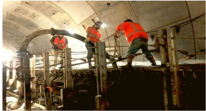
Reach 2 South Tunnel Walkway Construction
