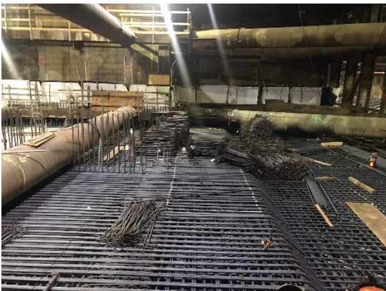
Station Entrance Concourse Level Roof Slab Rebar Installation at the Wilshire/Rodeo Station
