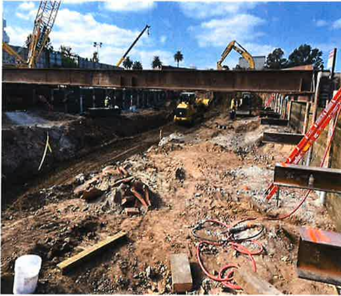
Westwood/VA Station Facing West - Excavation for Station Box and Level 1 Bracing
