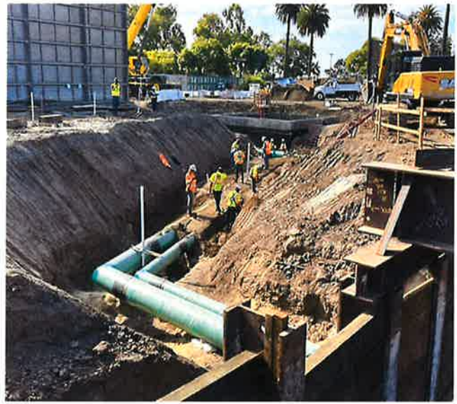
VA Steam Tunnel – Backfill Redundant Lines
