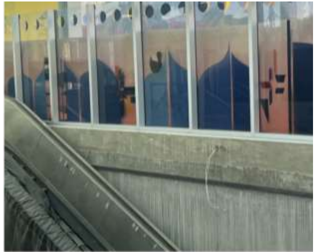
Wind barrier glass at Plaza Level West at Little Tokyo/Arts District Station
