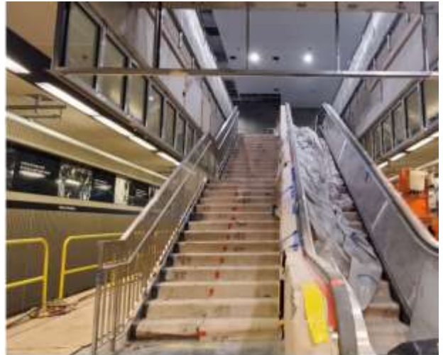
Platform Level at Historic Broadway Station
