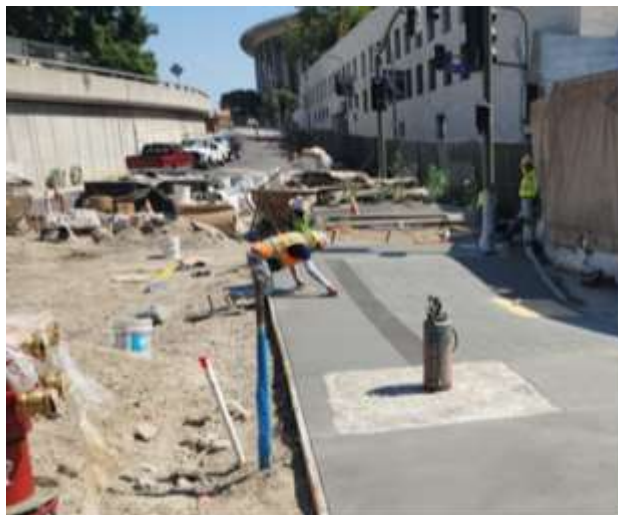
Sidewalk placement NE of Grand Av Arts/Bunker Hill Station Plaza Level
