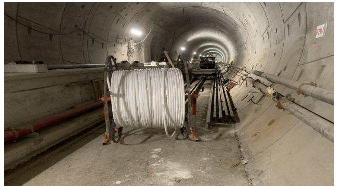
Reach 1 South Tunnel Communications Installation
