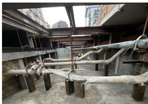
Backfilling Sewer and Storm Drain Bypass at the west end of Century City Constellation Station
