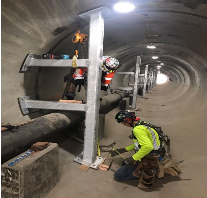
VA Steam Tunnel Relocation: Installing Pipe Racks
