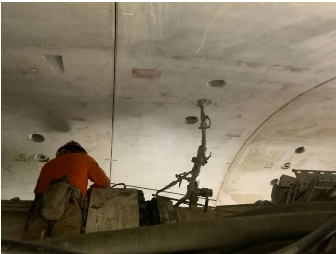
Tunnel: Secondary Grouting on Ring #1857
