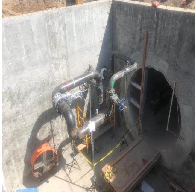
VA Steam Tunnel Relocation: Vault 200 Redundant Pipes Installed
