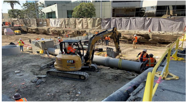
Weekend Decking Removal at Wilshire/La Cienega Station
