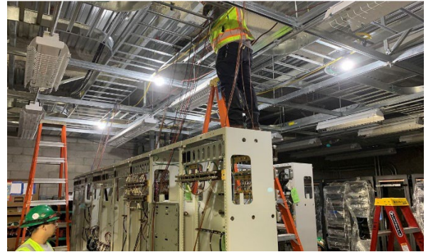
Automatic Train Control Work at Wilshire/La Brea Station
