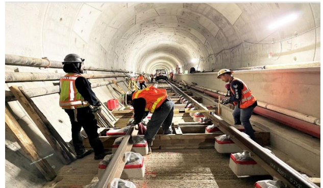
Reach 2 (BL) Track Installation
