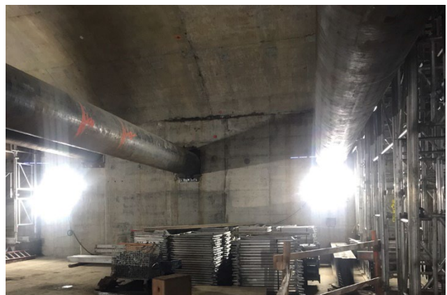
Falsework removal at the WRS concourse
