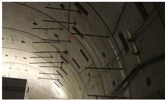
Installed Lances for Chemical Grouting at CP 36
