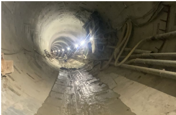
Cross Passage Tunneling activities
