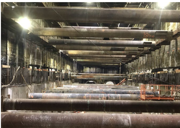
Restrutting at the Wilshire/Rodeo Station Box
