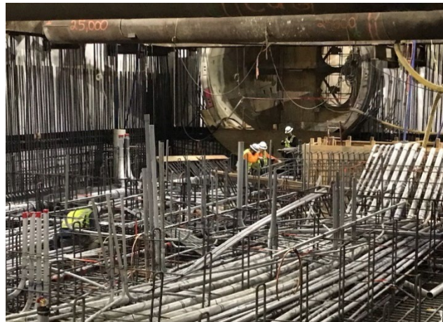
Conduit and Rebar Installation at WRS (West Hammerhead)
