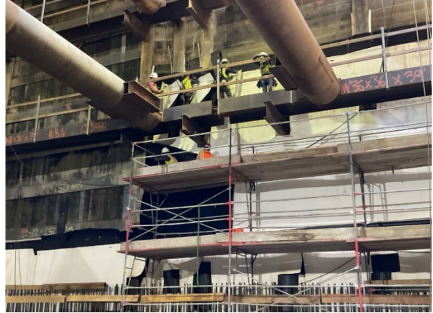
Waterproofing at CCCS (North Wall)
