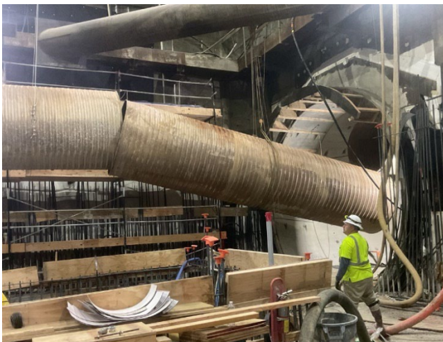
Re-establishing Ventilation for BR Reach 4 at WRS
