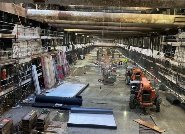
Strut Removal Looking West at CCCS
