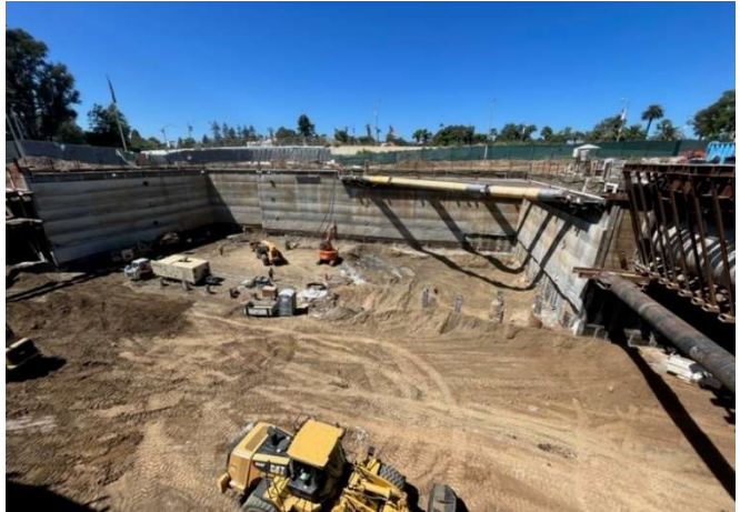
Westwood/VA Station Entrance: Installation of Level 4 Tiebacks & Shotcrete Lift #6
