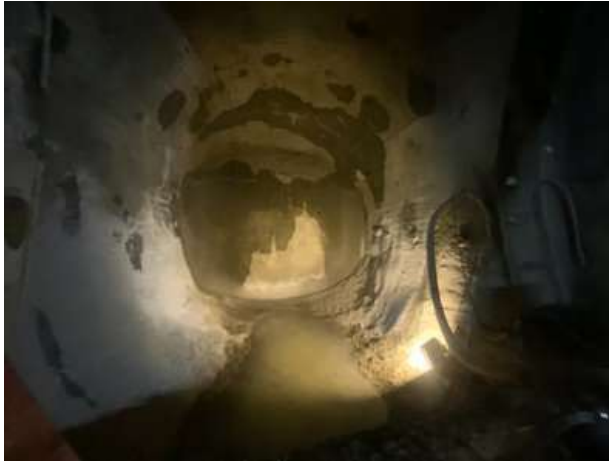
Cross Passage CP-53 in BR Tunnel: Completed Excavation and Initial Lining
