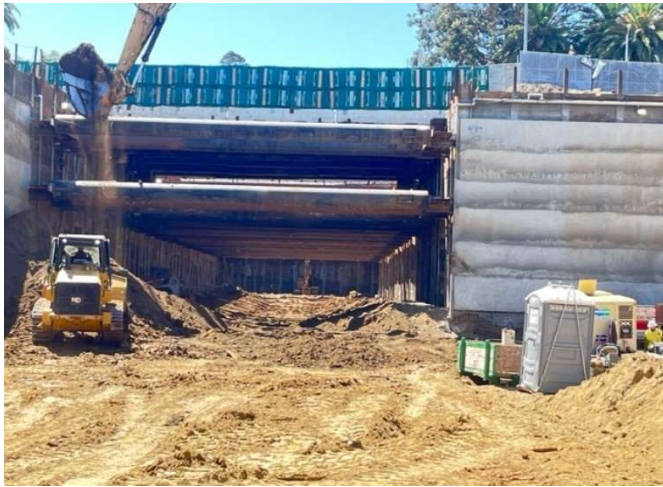
Westwood/VA Station: Excavation and Lagging for Level 3 West Bonsall
