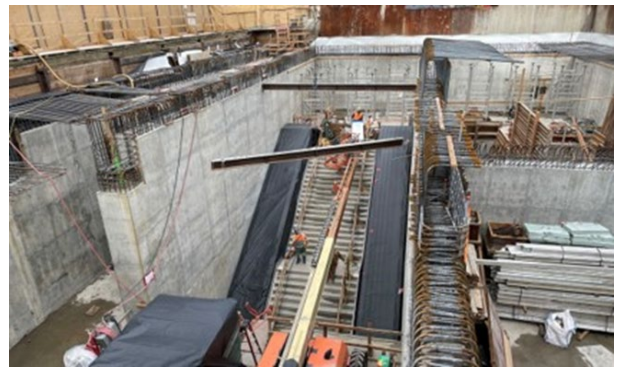
Wilshire/La Cienega Station Entrance Plaza Steel Supports
