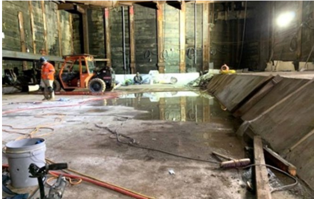
Wilshire/Western Interface Chamber Roof Water Protection Membrane Installation
