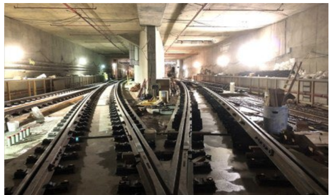
Wilshire/La Cienega Station Double Crossover Installation
