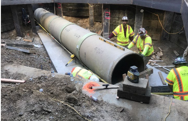
CCCS Storm Drain Pipe Installation
