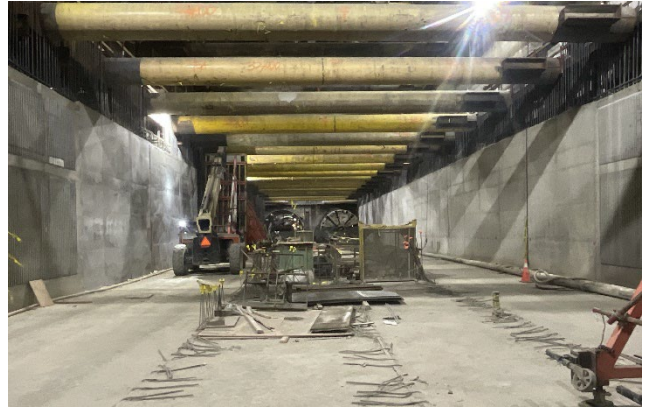
CCCS Westside Platform Level Exterior Wall Progress
