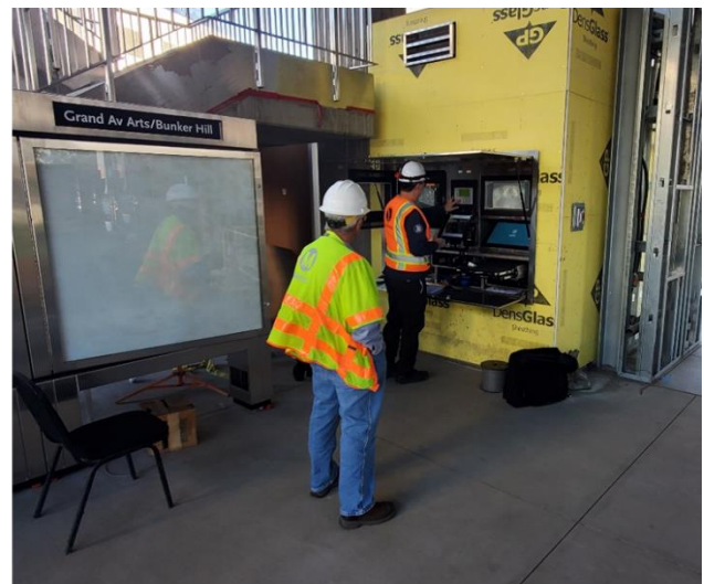
Fire alarm testing within station of Grand Av Arts/Bunker Hill Station
