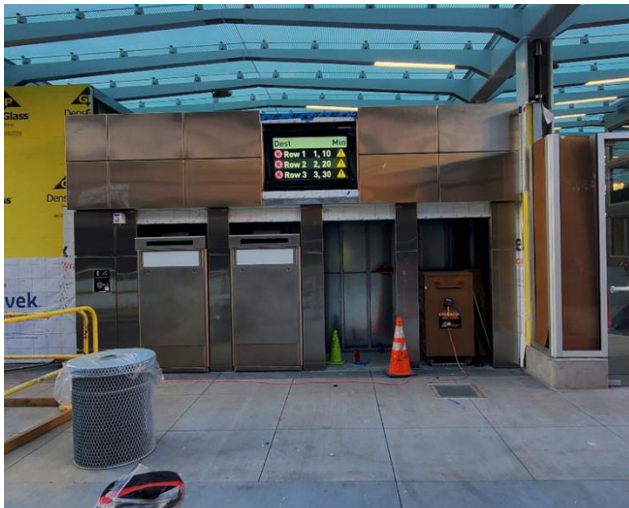
TVM installation at East Plaza level of Historic Broadway Station
