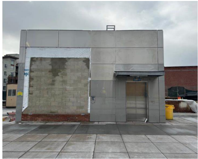
Headhouse cladding progress of Little Tokyo/Arts District Station
