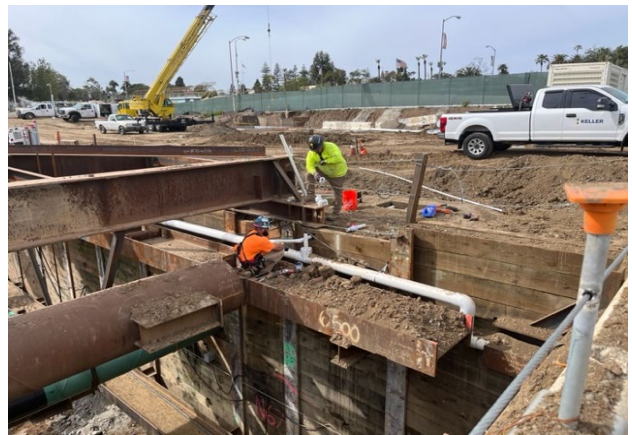
Westwood/VA Station Dewatering System Laterals Installation
