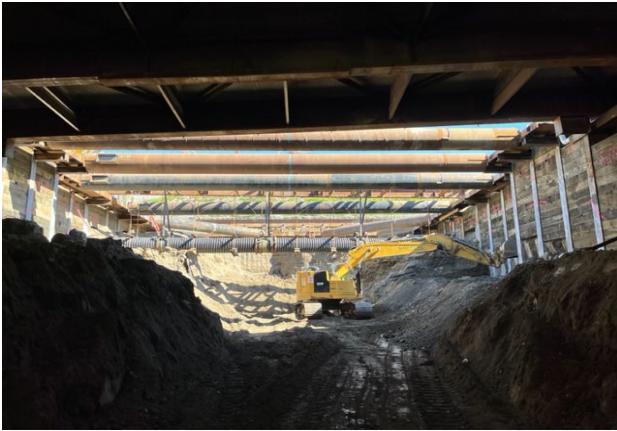
Westwood/VA Station: Under (Under I-405) Excavation Ongoing
