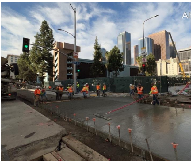
Concrete placement at west Spring St
