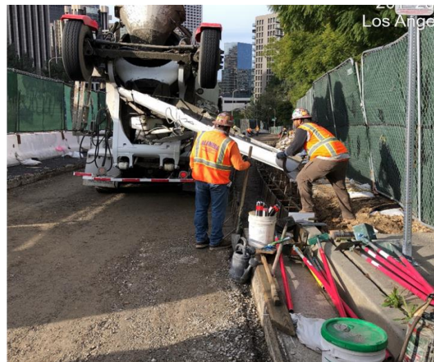
Curb and gutter placement at southbound Flower St
