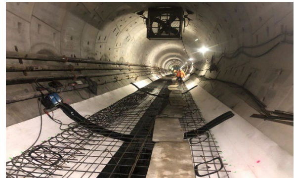
Reach 4 (BR) Invert Construction
