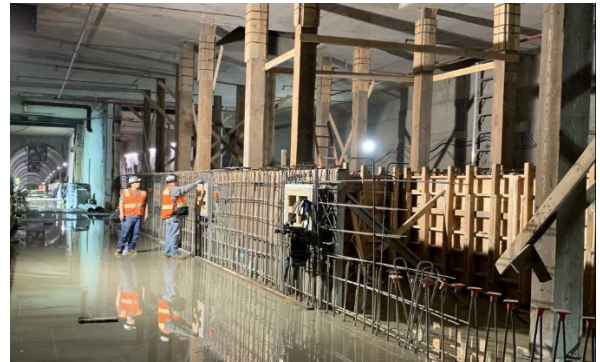
Wilshire/La Cienega Station Platform Wall Construction
