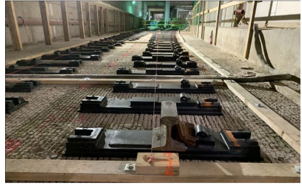
Crossover Plate Installation at Wilshire/La Brea Station
