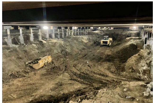
Westwood/UCLA Station - Level #1 Excavation and Installation Lagging Under Street Decking
