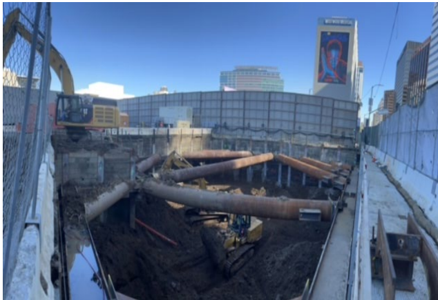
Westwood/UCLA Main Entrance – Level #1 Excavation and Lagging Installation
