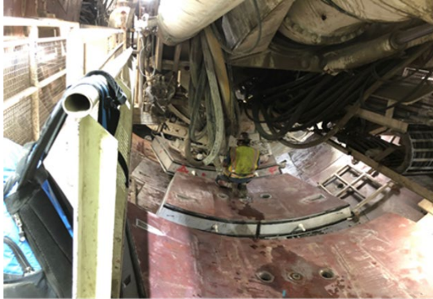
BL Tunnel Special Seismic Ring Erection
