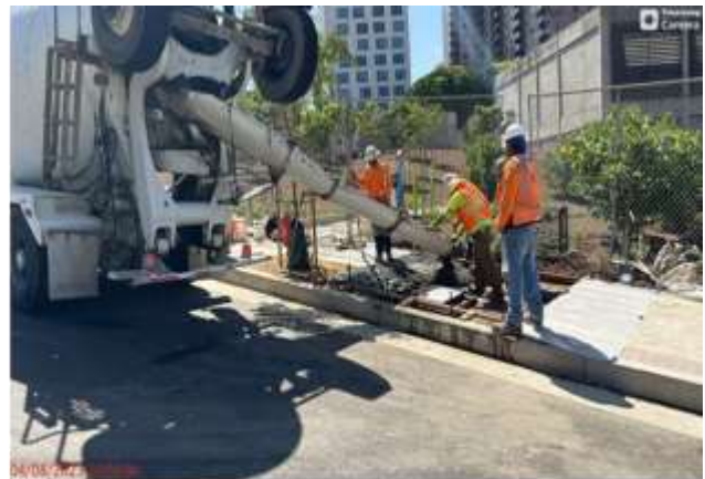
Placed concrete for remaining portion of sidewalk along NB Flower St
