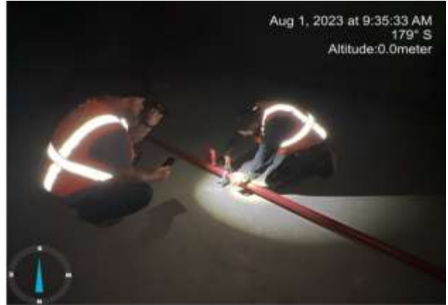
Completing fire suppression placement at the SEM Plenum
