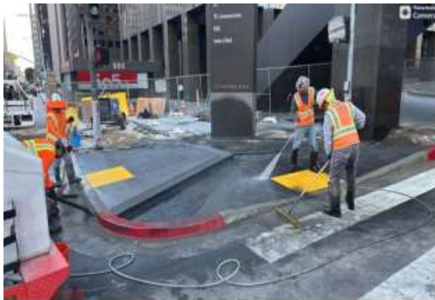
Concrete placement for 5 & Flower St at SW corner
