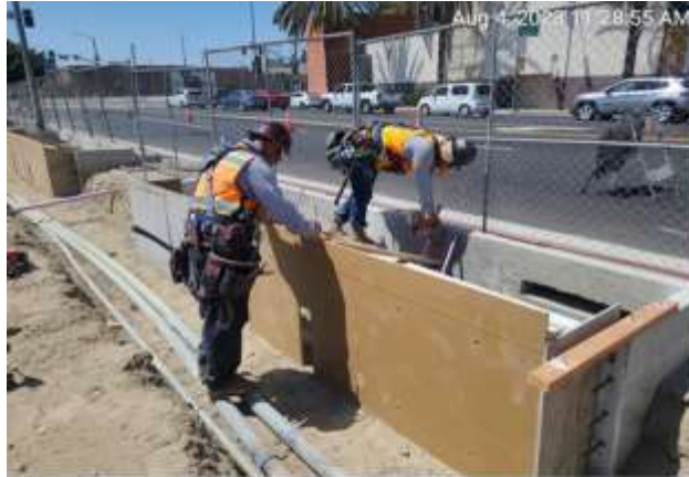
Building forms for bioswales modifications on Alameda
