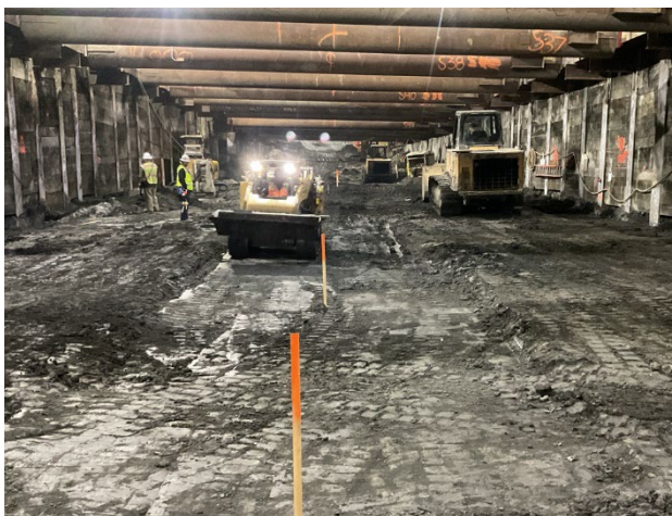
Grading at CCCS Bottom of Excavation
