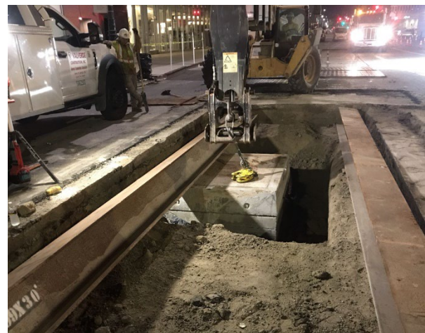
SCE Excavation (West) WRS Station Box
