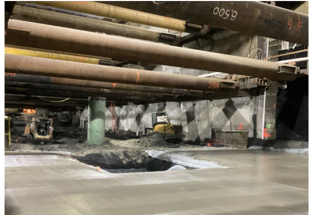
Capping Mud Slab at CCCS Invert
