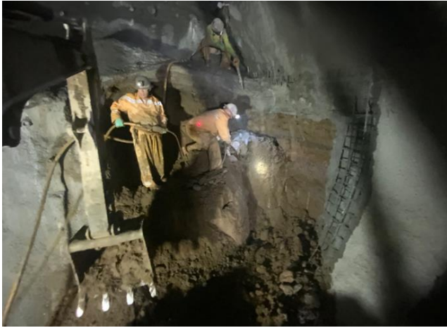
Cross Passage CP-54 in BL Tunnel: Excavation at Bench
