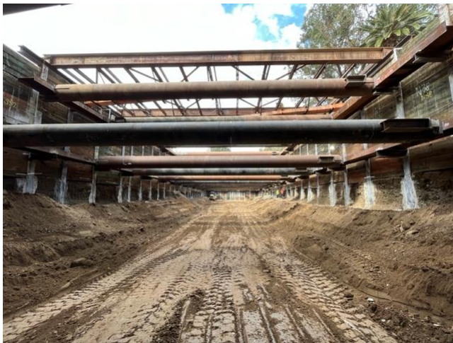
Westwood/VA Station: Excavation and lagging for Level 3.
