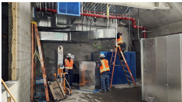
HVAC Ductwork Installation at Wilshire/Fairfax Station
