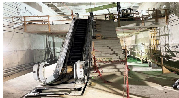
Escalator Installation at Wilshire/La Cienega Station
