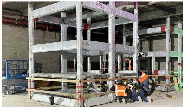
Elevator Frame Installation at Wilshire/La Brea Station
