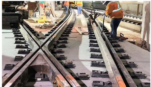
Track Crossover Construction at Wilshire/La Brea Station
