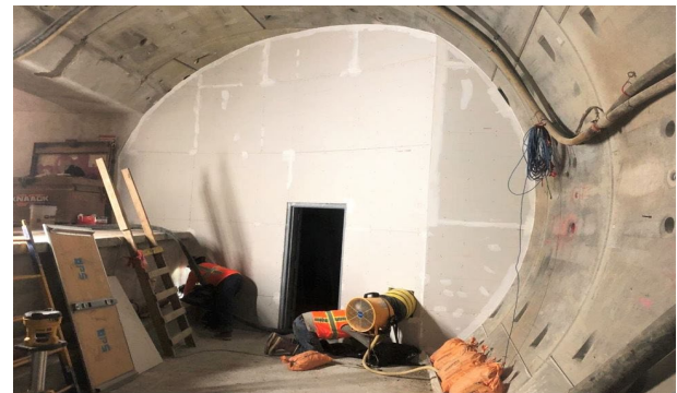
Reach 4 BR Tunnel Bulkhead Wall Installation
