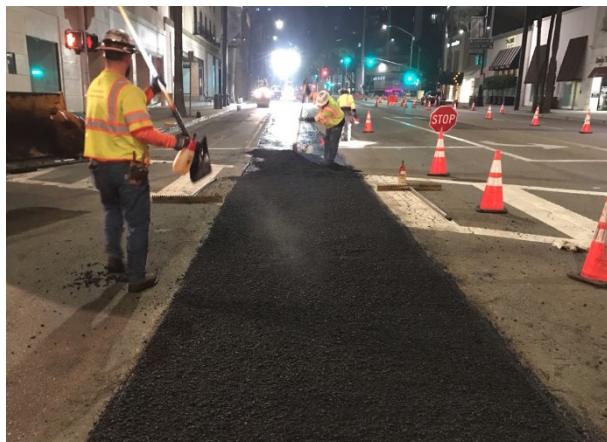
SCE Trench Restoration on Wilshire Blvd (WRS)
