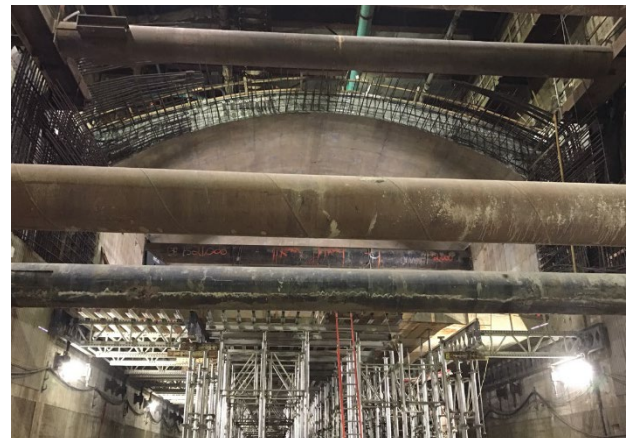
Falsework removal at the WRS Station Box
