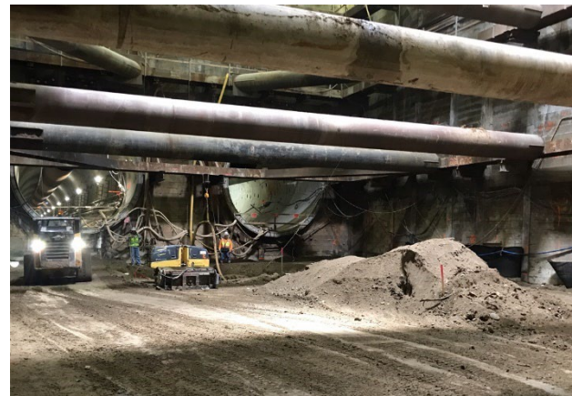
Preparation of Subgrade at the WRS Station Box
