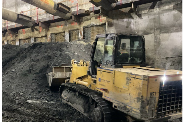
Excavation (West Side) at CCCS
