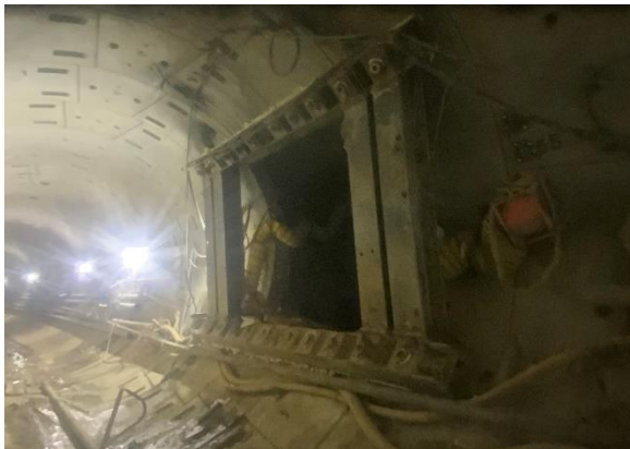
Cross Passage Excavation
