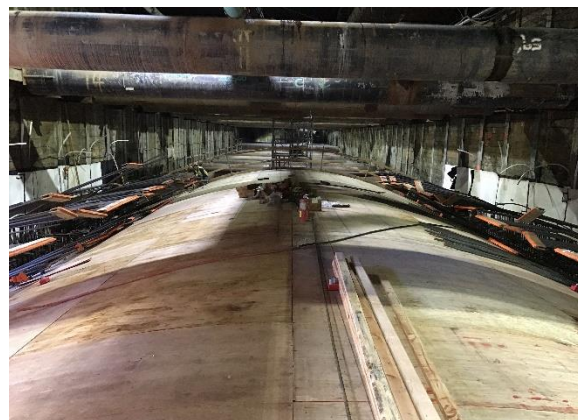
Concourse Level Roof Rebar Installation at the Wilshire/Rodeo Station Box
