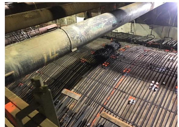
Concourse Level Roof Rebar Installation at the Wilshire/Rodeo Station Box
