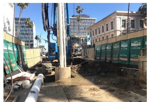
Dewatering Well Activities in Beverly Hills
