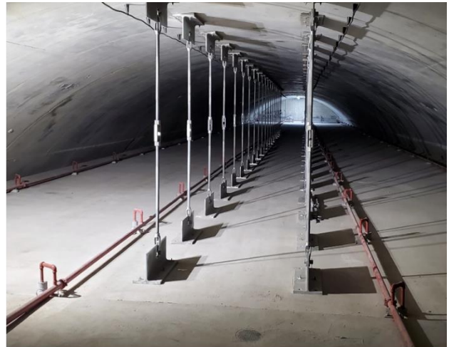
SEM Plenum slab support system
