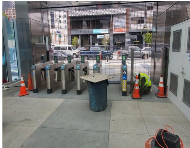
Emergency Swing Gate at west entry portal at Historic Broadway Station
