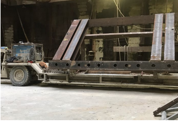
Preparing for Cross Passage Picture Frame
