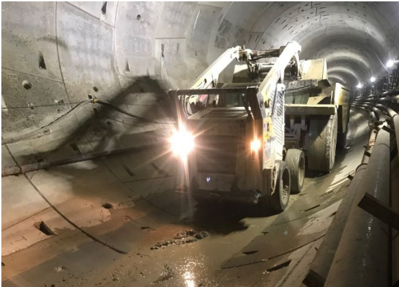
BL Tunnel Mucking for Cross Passage Excavation
