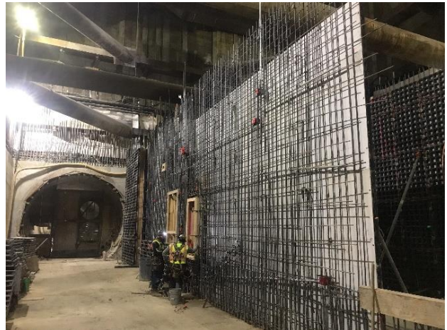
WRS West Module Interior Walls Formwork and Rebar
