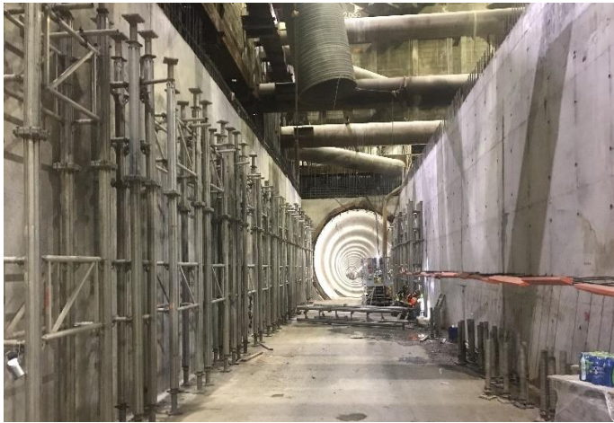
WRS Falsework for Concourse Level Slab East
