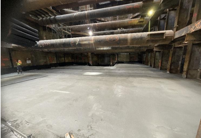
CCCS Capping Mud Slab at Entrance
