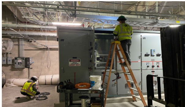
Switchgear Installation at Wilshire/La Cienega Station
