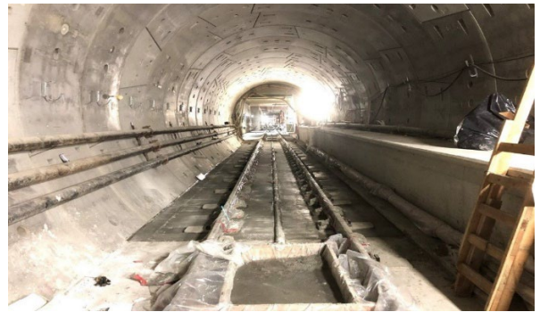
Reach 4 (Tail Track) Track Concrete Infill
