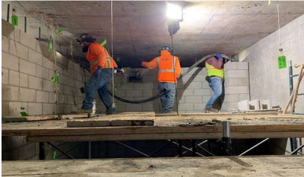
Masonry Work at the Wilshire/Western Interface Chamber
