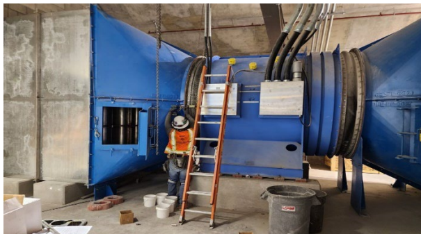
Ventilation Fan Installation at Wilshire/Fairfax Station
