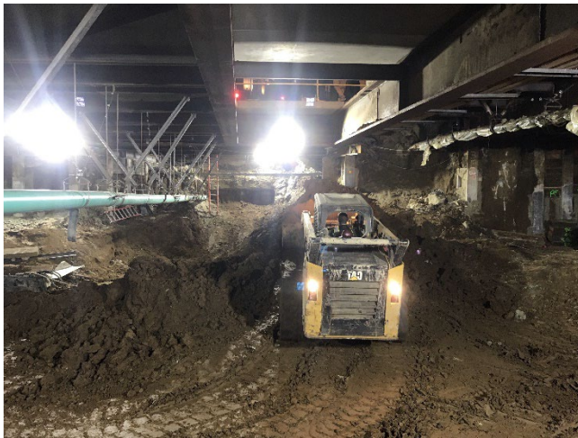
WRS Grating #9 Excavation - South Beverly Appendage
