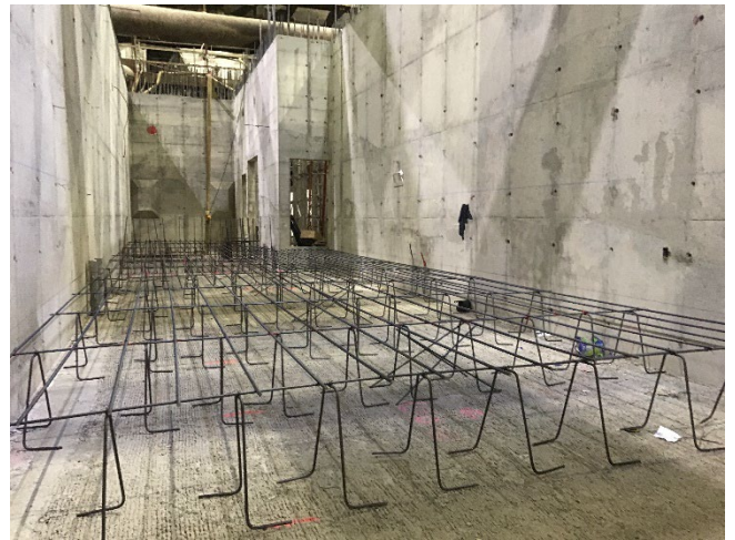
WRS Interior Slab Rebar - East Hammerhead
