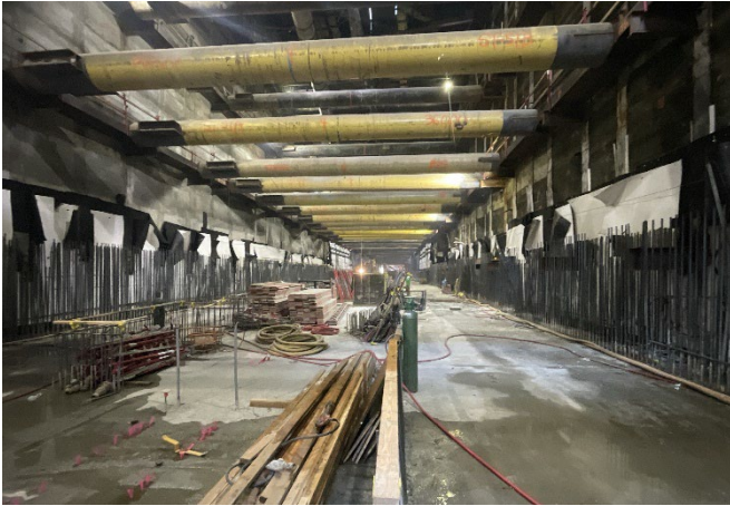
CCCS Platform Level Walls Looking East
