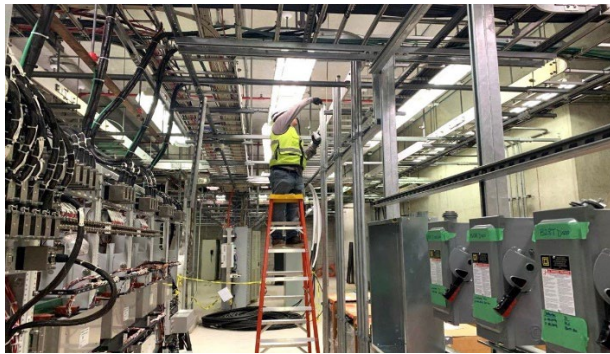
Wilshire/Western Station TC&C Room Conduit Installation
