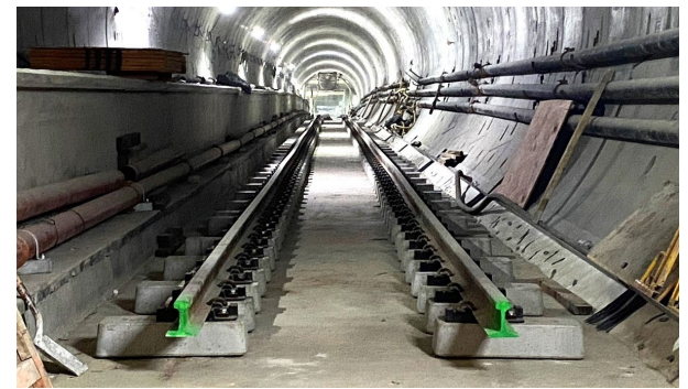
Reach 4 (Tail Track) Track Installation
