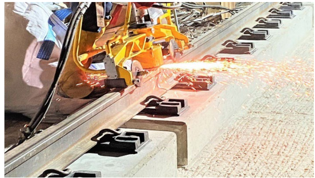
Rail Weld Grinding at Wilshire/La Brea Crossover
