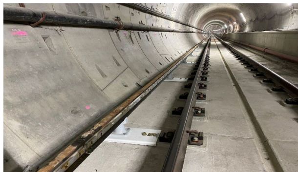
Reach 3 Contact Rail Installation
