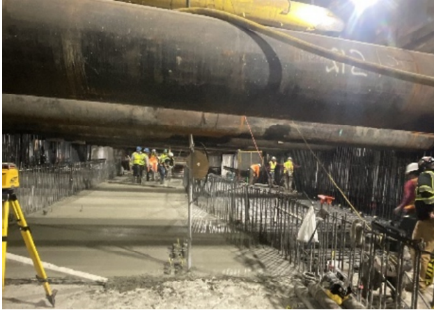
Placing Concrete at CCCS Invert
