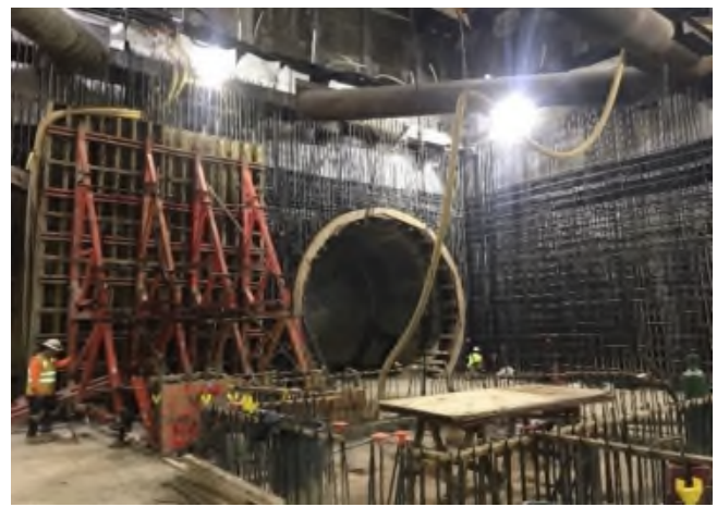
End Wall Formwork at WRS (west end)
