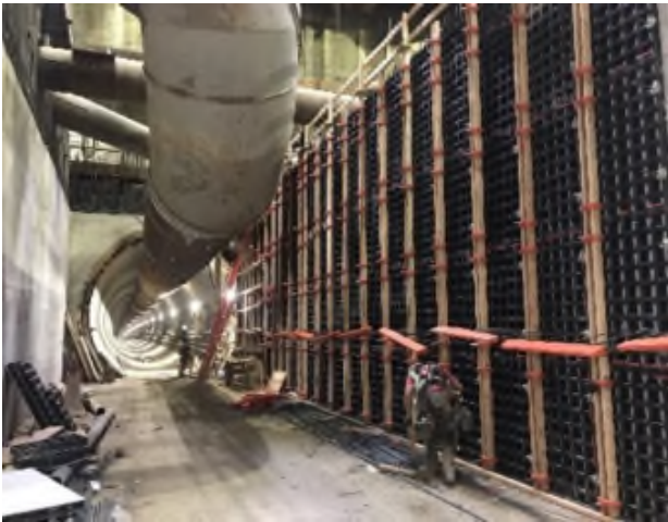
Interior Wall Formwork at WRS (east end)
