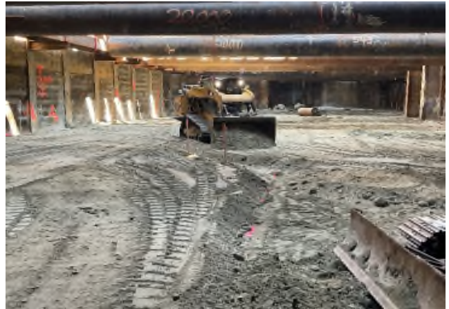
Grading at CCCS Entrance
