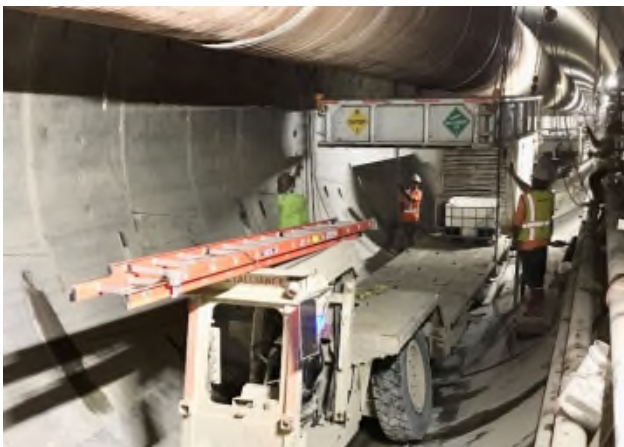
Reach 4 Refuge Chamber Removal
