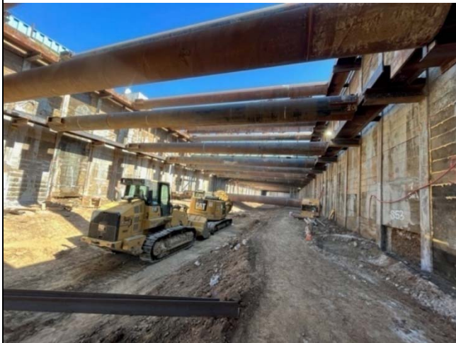
Westwood/VA Station: Excavation Support Bracing at Level 3, West of Bonsall
