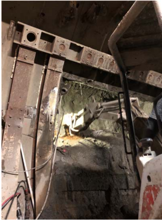
Cross Passage CP-52 in BL Tunnel: Excavation and Initial Lining Installation
