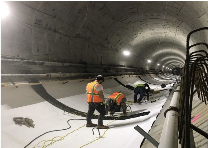
Reach 5 BL Tunnel Invert Waterproofing
