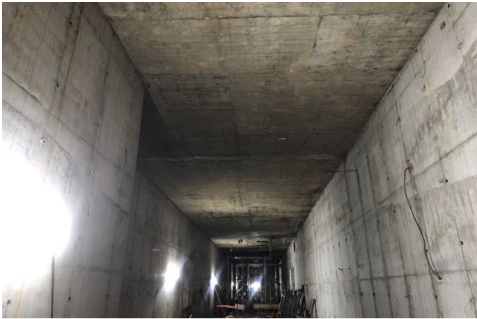
WRS East Concourse Level Slab Falsework Removal
