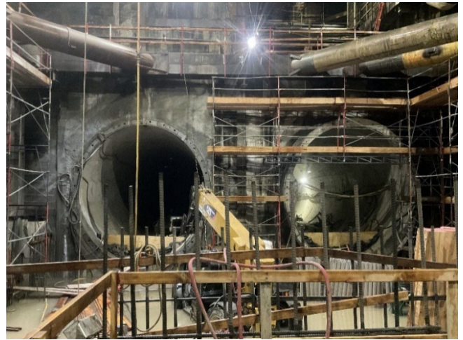
CCCS West Endwall Waterproofing Membrane Scaffolding
