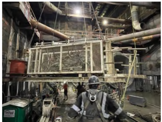
BL TBM Gantry Extraction from Century City/Constellation
