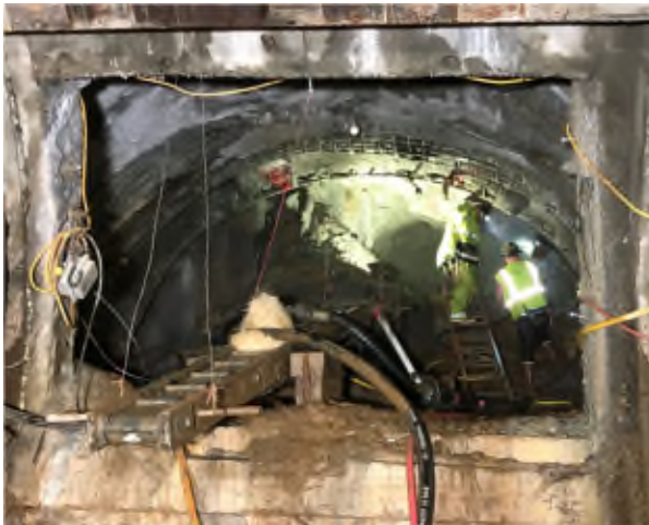
BL Tunnel Cross Passage CP-52 Excavation at the Top Heading
