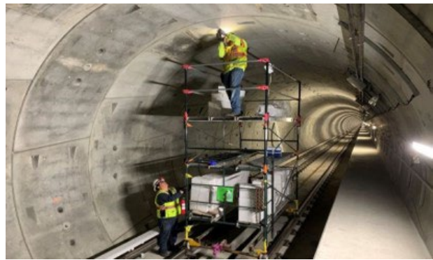
Reach 1 Tunnel BL Radio Cable Support Installation
