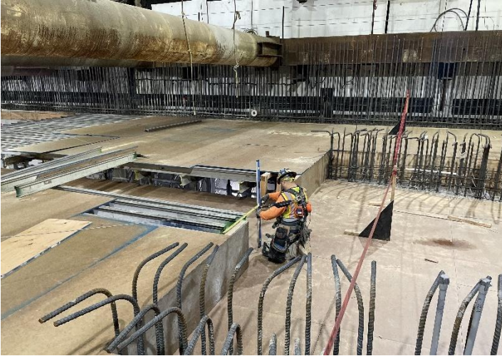
CCCS Falsework at CLS-4
