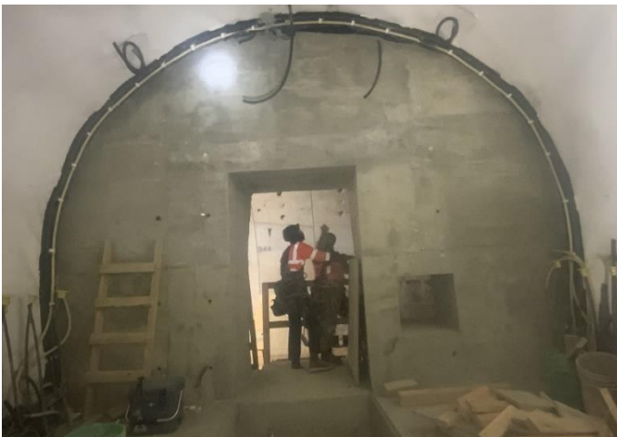
CP-35 Finished Bulkhead Inside
