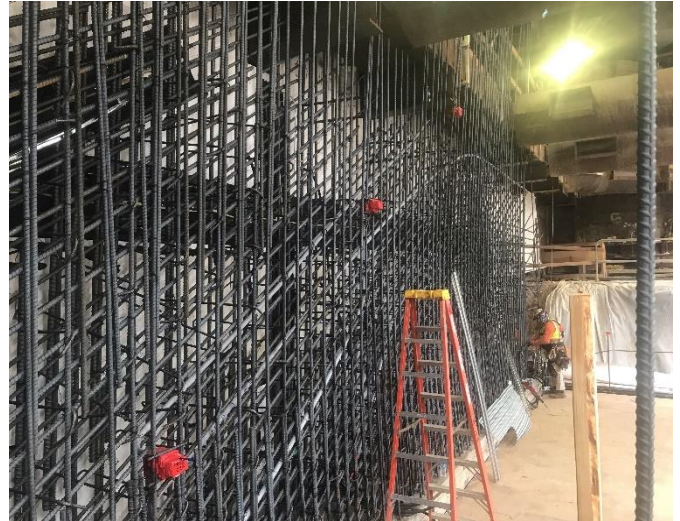
WRS Station Box Exterior Wall Rebar
