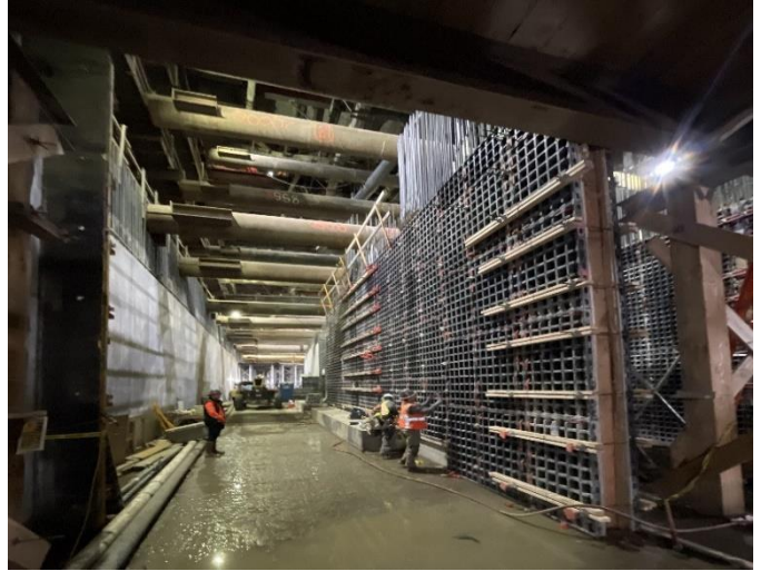
CCCS Stripping at Interior Walls
