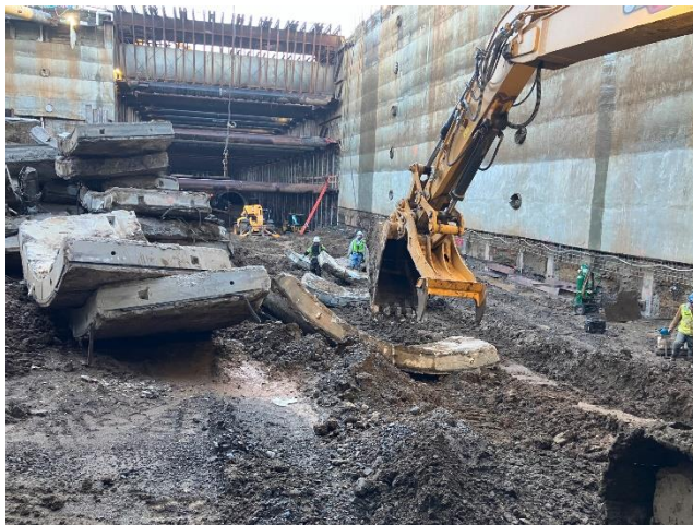
Westwood/VA Hospital Station: Removal of Tunnel Segments Looking East
