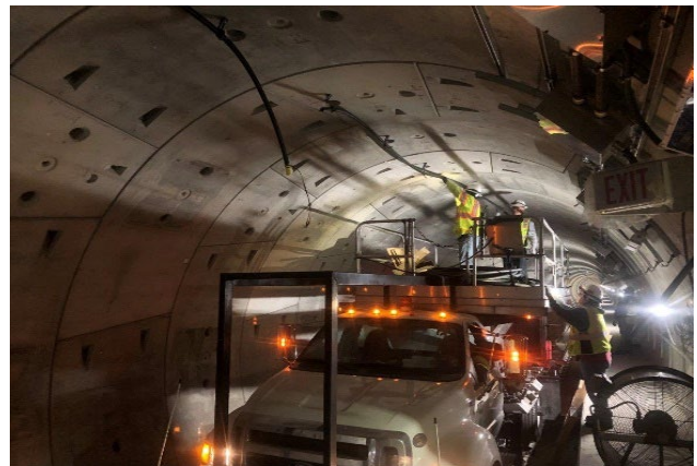
Reach 1 Tunnel Radio Wire Installation
