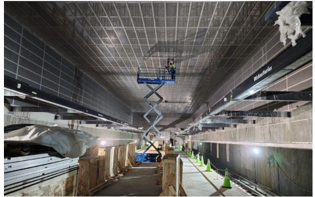
Wilshire/Fairfax Station Radio Cable Supports Installation
