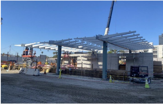
Wilshire/La Brea Station Main Entrance Canopy Installation
