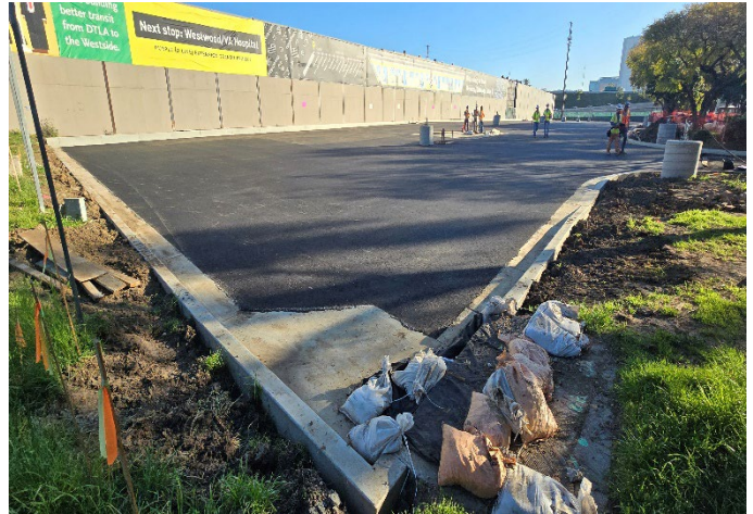
VA Parking Structure: Lot 42 Asphalt Paving Completed
