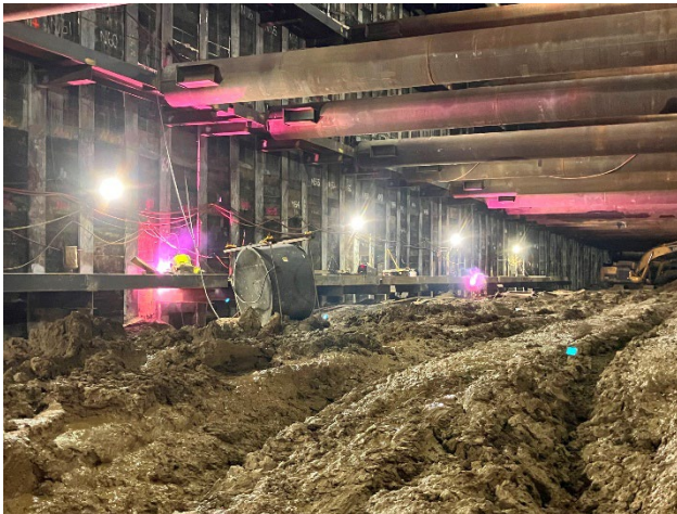
Westwood/UCLA Station: Welding of BL4 Waler Support on the North Wall
