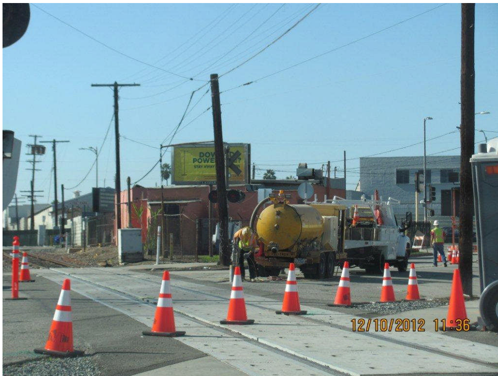
Utility location at 67 th Street.
