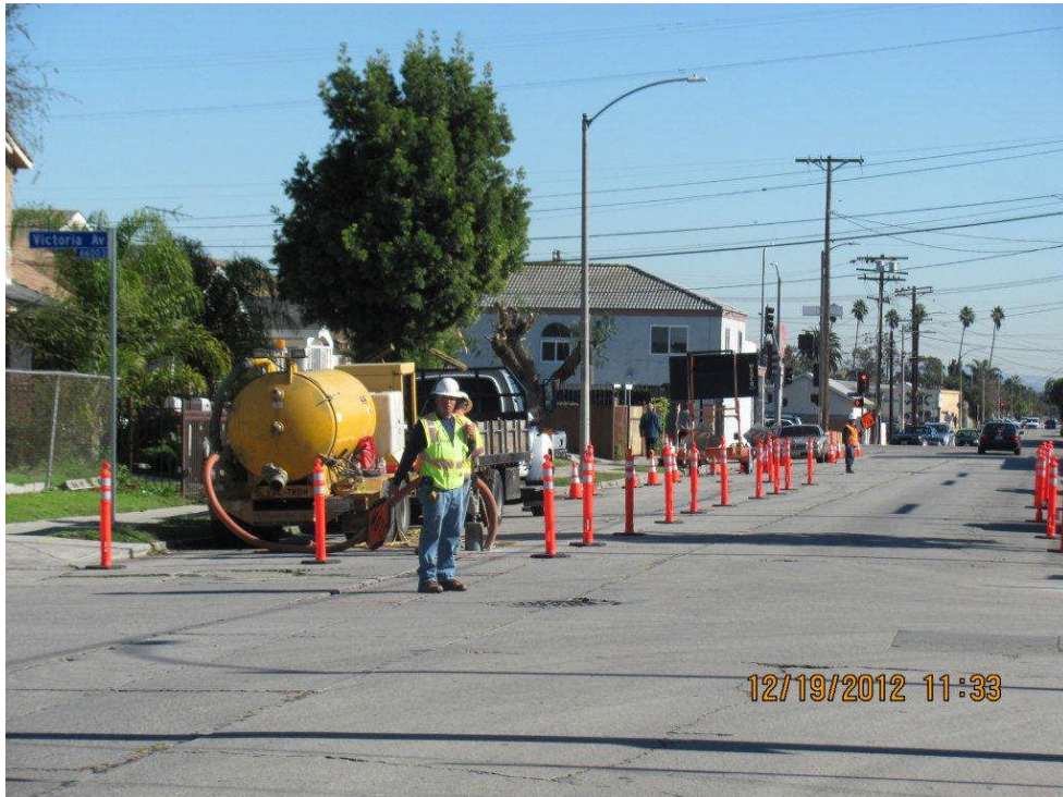
Traffic Control at Victoria Street.
