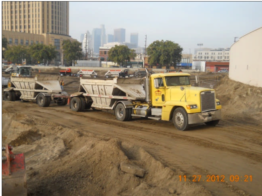
Removal of hazardous soils.
