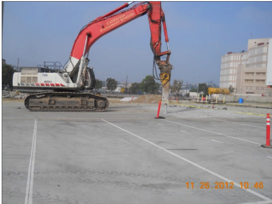
Demolition of surface pavement.
