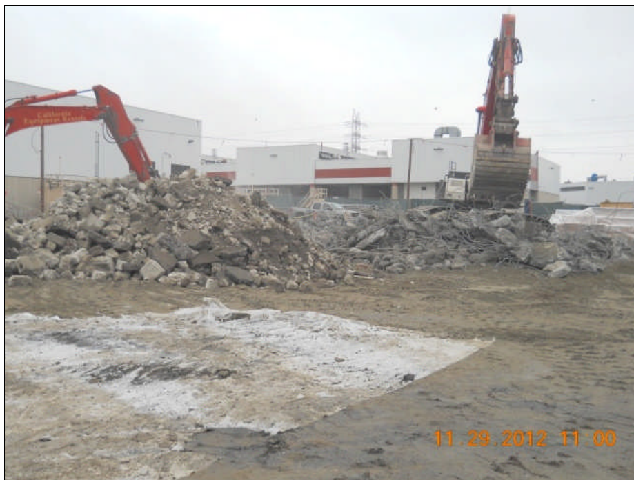
Demolition of surface pavement.
