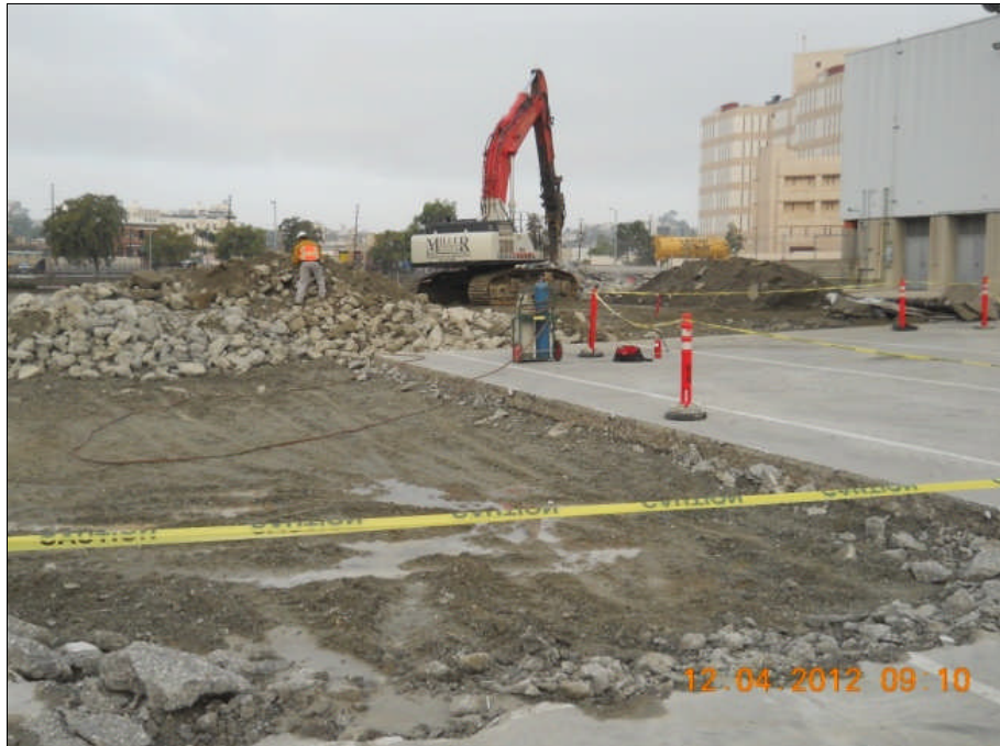
Demolition of surface pavement.
