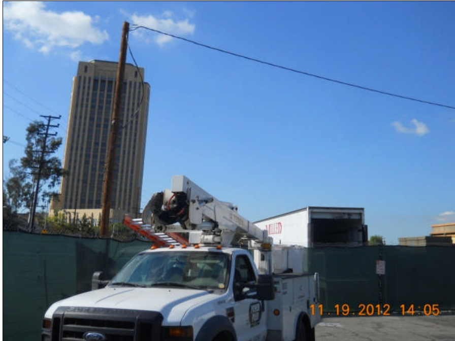
Temporary power pole installation.
