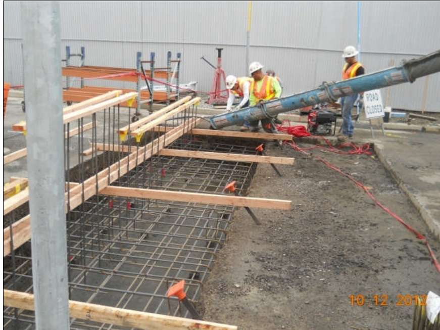
Construction of concrete mock up.
