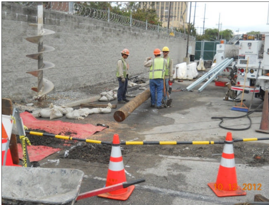
Installation of temporary power poles.
