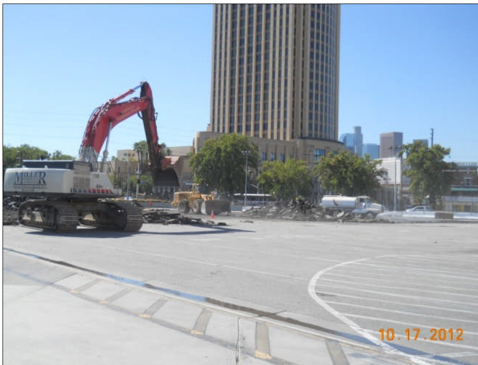
Demolition of existing parking area.
