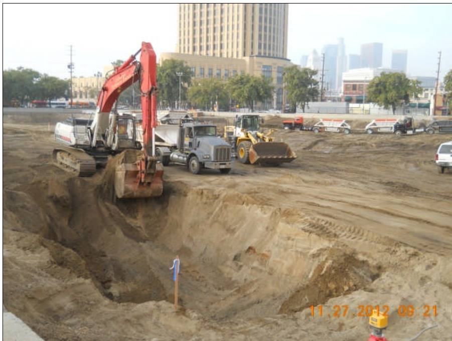
Removal of hazardous soils.
