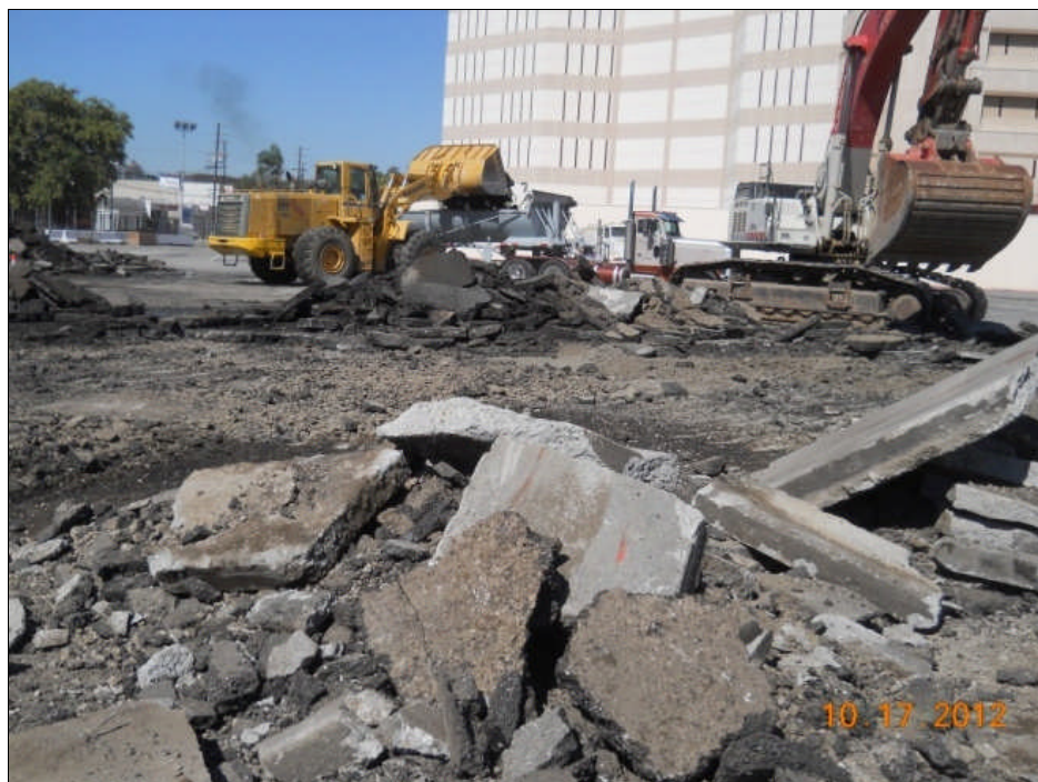
Demolition of asphalt pavement.
