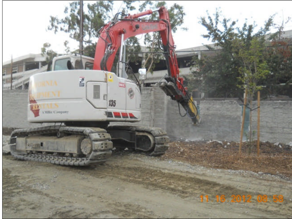
Demolition of site walls.
