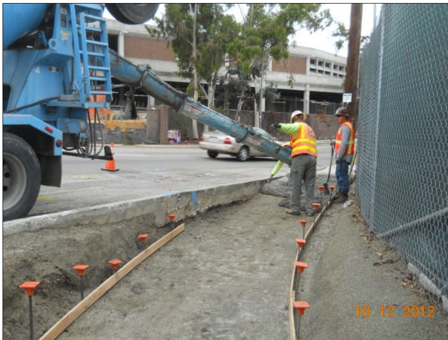
Placement of concrete walkway.
