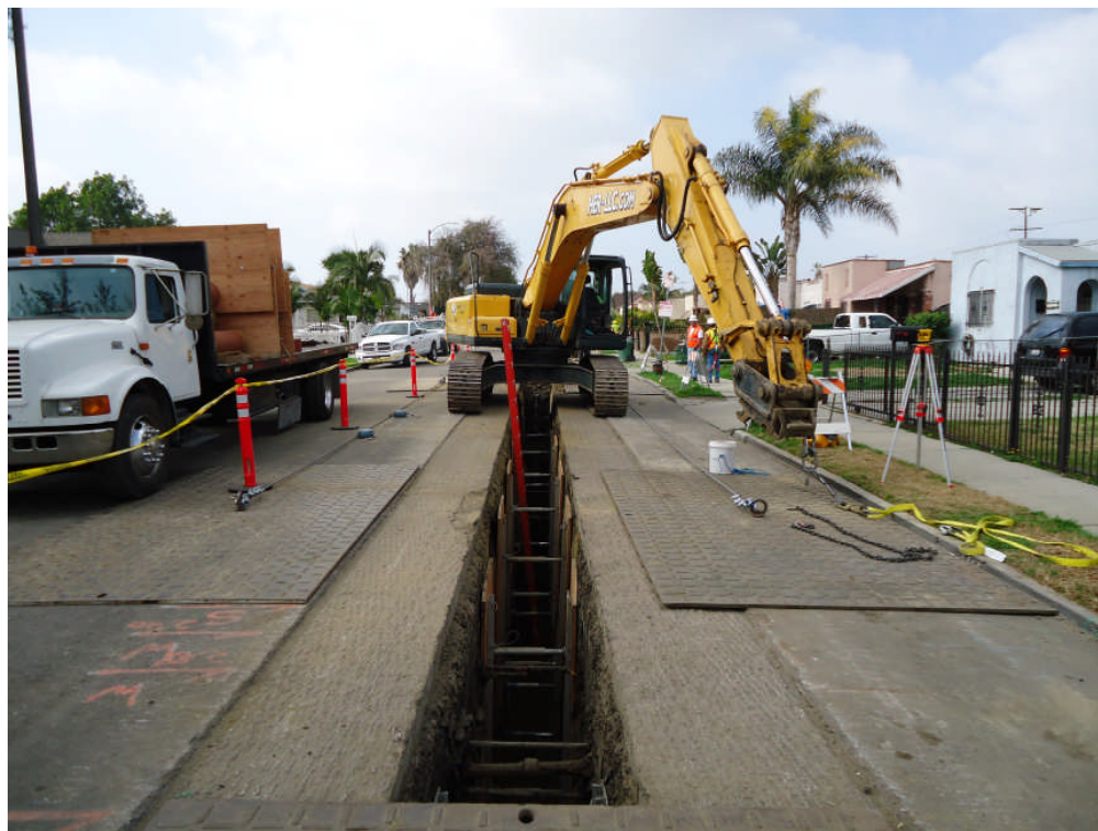
Trench work at 59 th Street.
