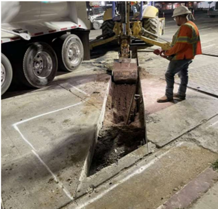
Starting A18 lateral excavation along Van Nuys Blvd
