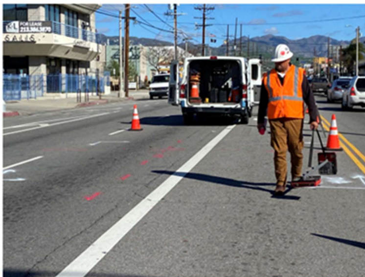
Operation to mark Phase II Hazardous Materials Boring Location DYE21-30 and check for Underground Utility Conflict
