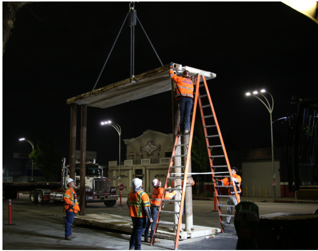
W.A. Rasic crew assembled second shoring box for Vault 6940
