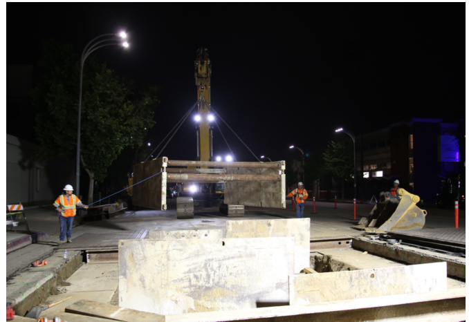
Second shoring box for Vault 6940 is transferred near the trench
