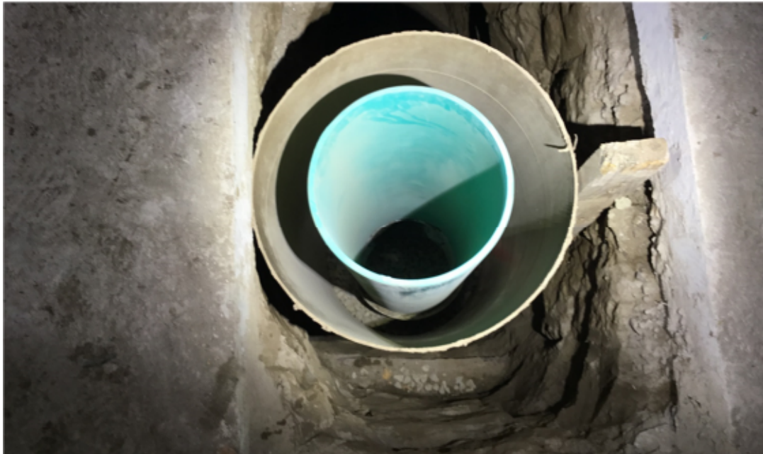
WA Rasic completed installation of 12" vents on Vault 6834
