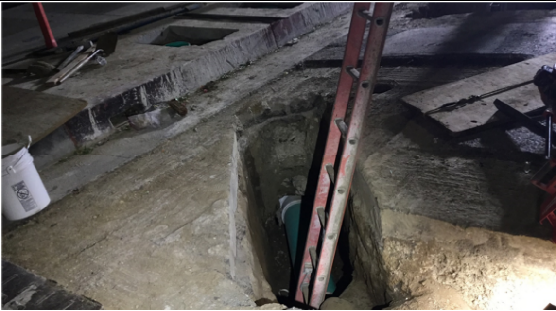
WA Rasic: Completed installation of 12" vents on Vault 6834
