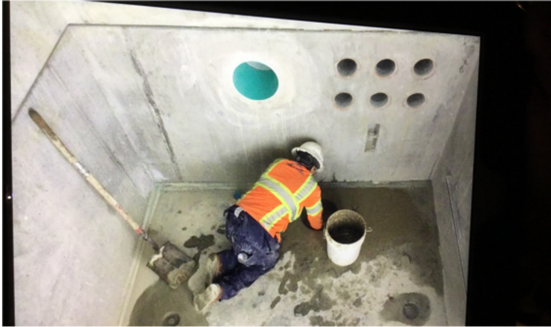
WA Rasic grouting and patching inside Vaults 6834, 6900 and 6940
