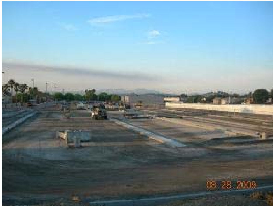
DSCN4277 C0941 looking south.
